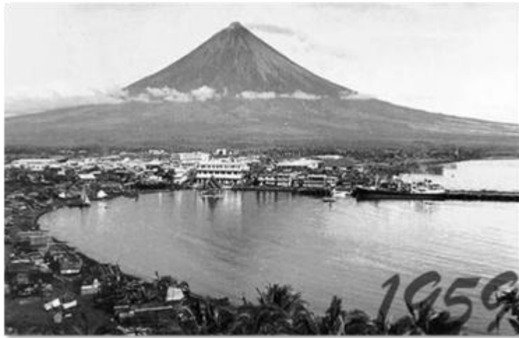
Fig. 19. 1959 phot of the Legazpi Port Source: Here in Albay webpage
