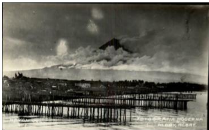
Fig. 11. Construction of the pantalans in Legazpi Port, during the 19 th century Source: Legazpi City Museum
